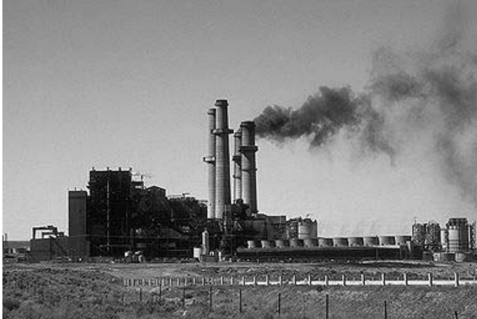
Figure 50. San Juan Generating Station in 1987. (reproduced with permission of G. Donald Bain; photo courtesy of The Geo-Images Project, Department of Geography, University of California, Berkeley, http://GeoImages.Berkeley.EDU )
