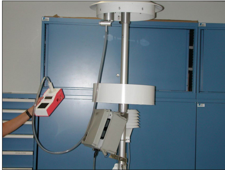
Figure 10.8 Flow audit device connected to SCC inlet.
