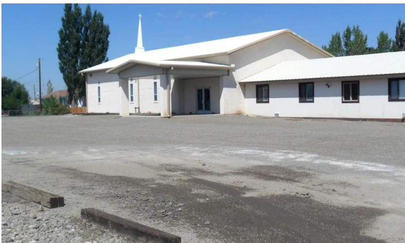
Figure 82: Site H as of August 2013 (CDPHE 2013)
