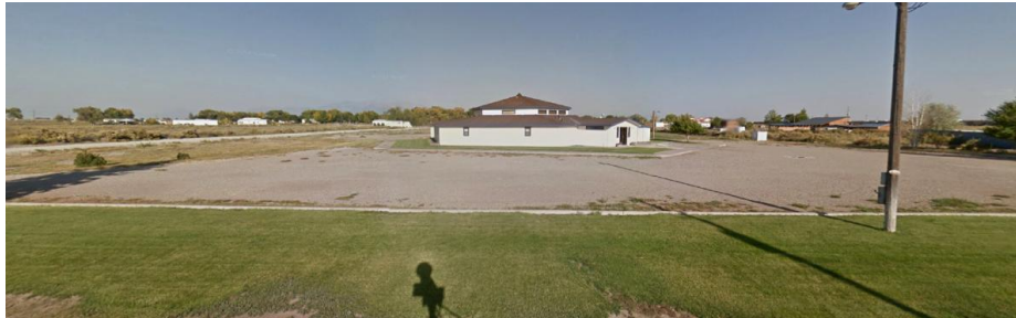
Figure 97: Site T (Google Image 2012)
