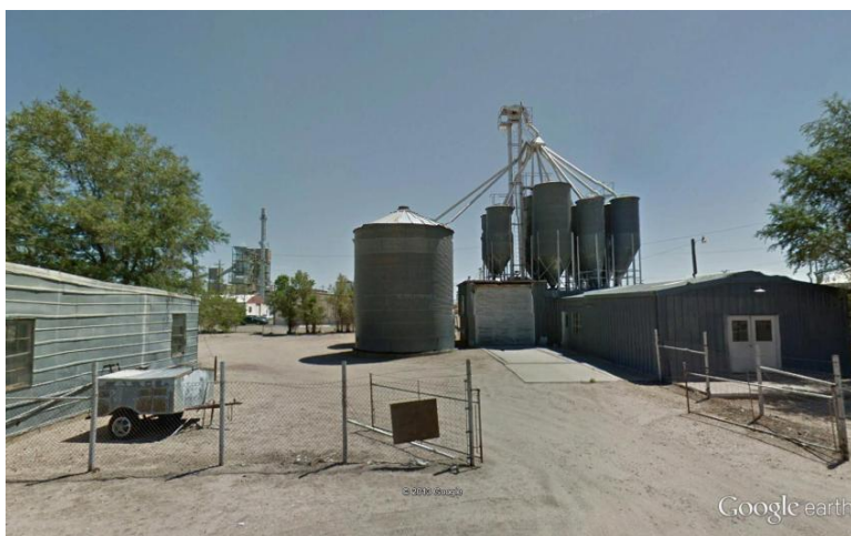
Figure 76: Feed Storage Company (Google Image 2012)
