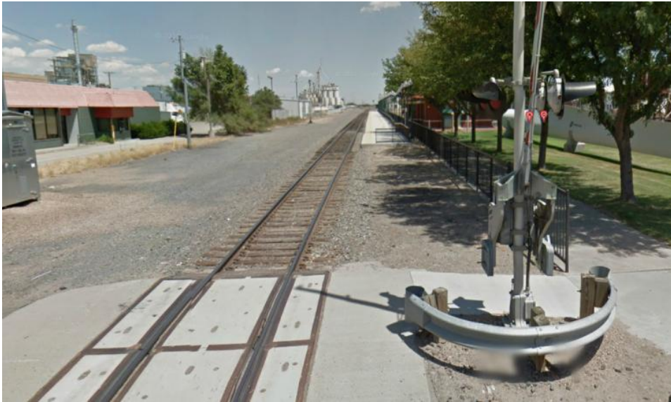
Figure 26: Railroad tracks with gravel on each side (Google Image 2012)
