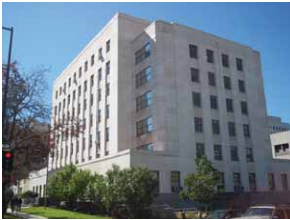
Zone 1 Exterior Facade: North and east elevations
