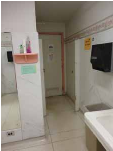
Fig. 3.1.C.6 Typical condition of terrazzo flooring in restrooms noted throughout.
