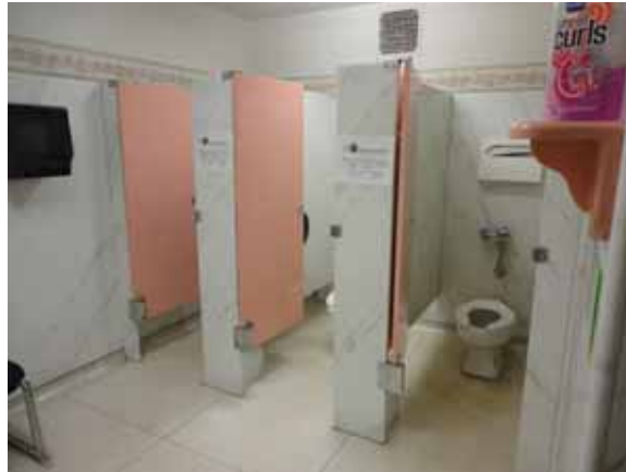
Fig. 2.1.C.2 Typical non-accessible bathroom stalls.
