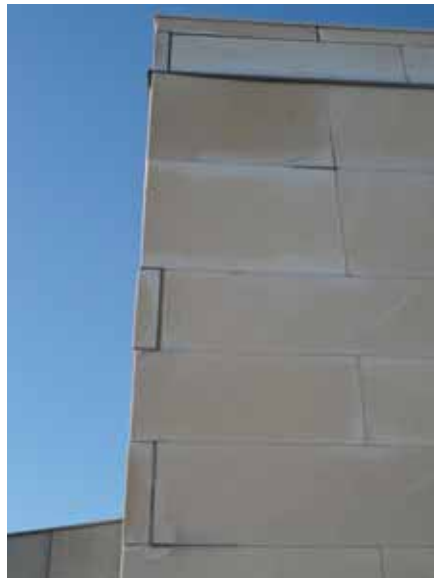
Fig. 2.1.A.4 Staining of marble panels cladding the Penthouse from previous repairs using an incorrect type of sealant.
