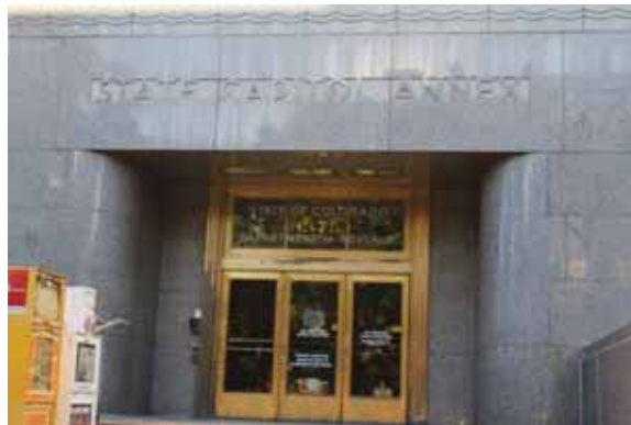
Figure 2.3.A.1 – Capitol Annex Sherman Street Entrance
