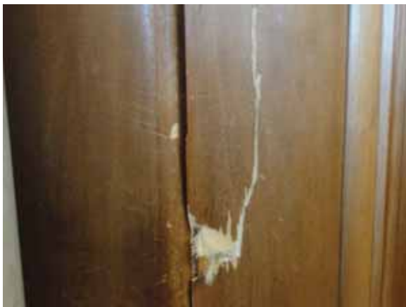
Fig. 3.7.C.3 Damaged wood wall paneling in Office 707 is part of an historic Hearing Room.
