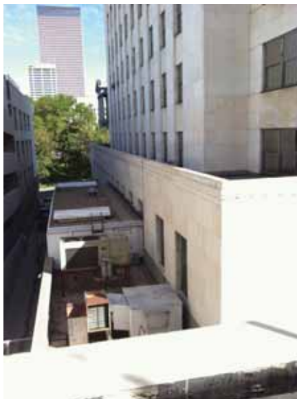
View of the Back/West alley between the Capitol Annex Building and the parking garage to the west, looking north
