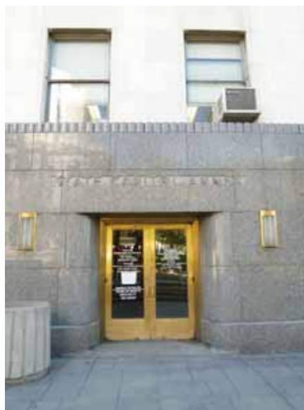
Zone 1 Exterior Facade: North entry with curved reveal at the door
