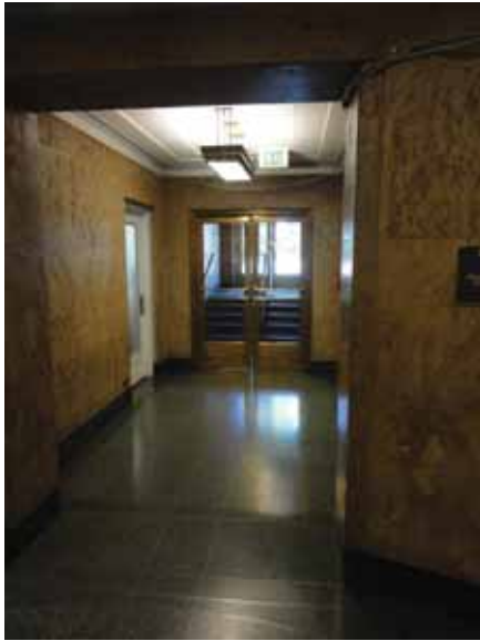
Fig. 2.1.B.2 The north 14th Avenue Entrance at the Basement Level has four steps up to grade and is therefore not an accessible entrance.
