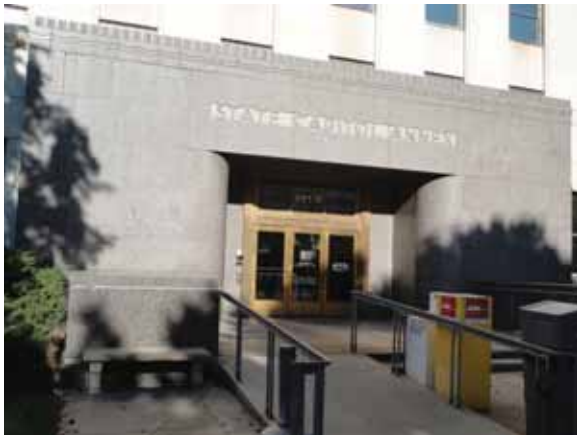
Front/East Sherman Street Entrance
