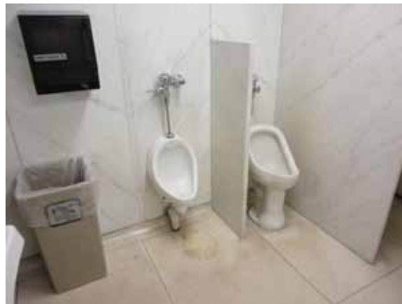
Fig. 3.1.C.4 Typical condition of terrazzo flooring in restrooms noted throughout.
