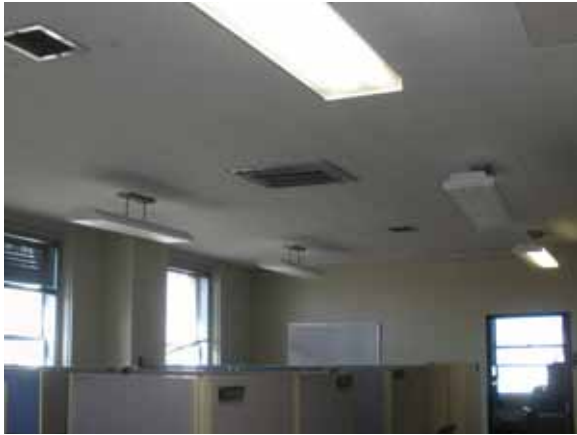
Fig. 2.4.A.1 - Old Light Fixtures
