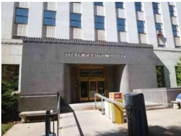
Zone 1 Exterior Facade: Granite clad east entry
