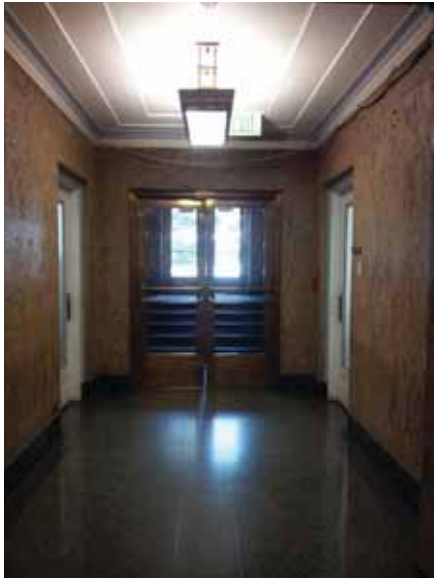
Zone 2 Interior Lobbies and Circulation: Basement corridor with typical finishes connecting to the north entrance
