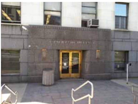
Side/North 14th Avenue Entrance
