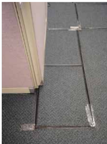
Fig. 3.0.1 Walkerduct Electrified Floor System: typical tombstone floor box covers found throughout the building.
