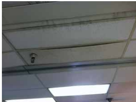
Fig. 3.4.C.1 2x4 acoustic ceiling tiles in generally poor condition.
