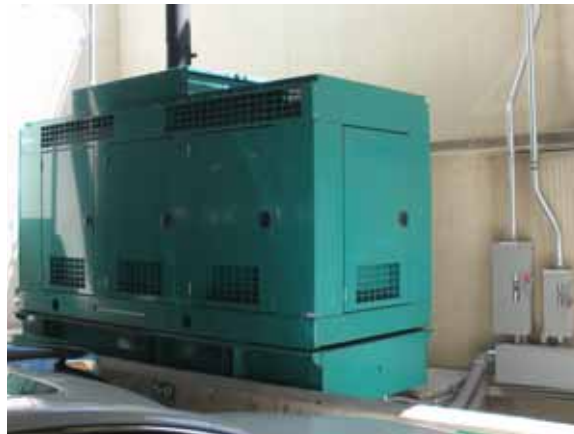
Fig. 2.4.A.8 - New emergency generator
