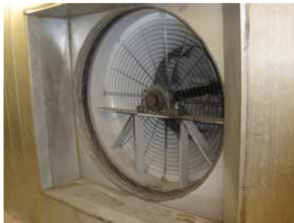
Fig. 2.4.A.10 - AHU Intake within built-up AHU
