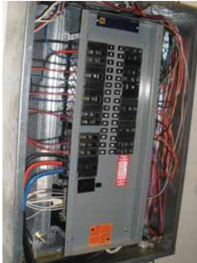
Fig. 2.4.B.3 - Missing panel cover
