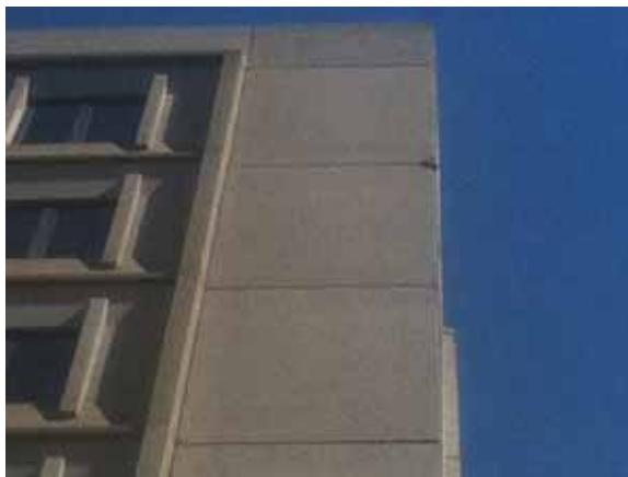
Fig. 2.1.A.2 Spalling at an exterior corner of the building.
