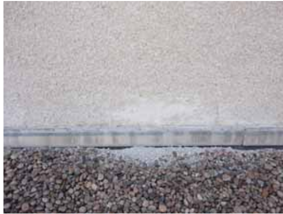
Fig. 2.1.A.5 Aggregate shedding from Penthouse panels.
