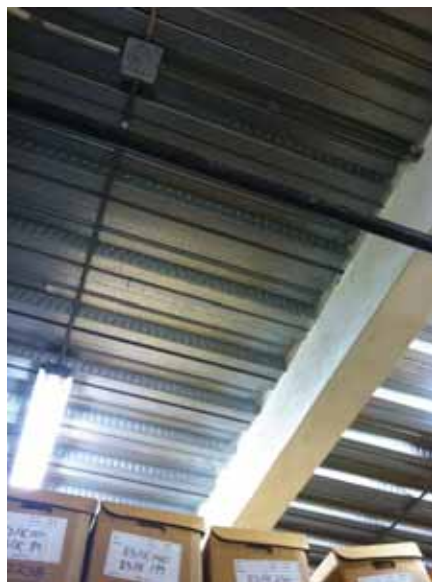
Fig. 3.10.C.1 The Division of State Archives and Public Records storage areas. Exposed metal decking at the ceiling with no fireproofing.
