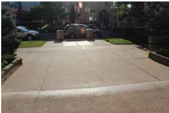
Figure 2.3.A.3 – Main Entrance Apron
