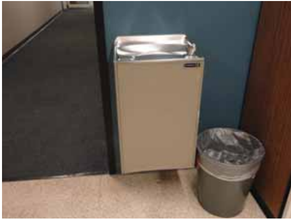
Fig. 2.1.C.3 Typical non-accessible drinking fountain found throughout the building.
