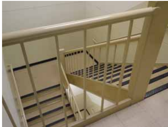
Fig. 2.1.B.2 Exit stair railings.
