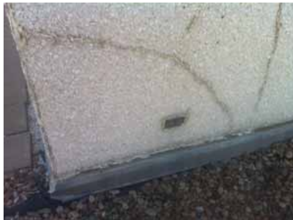
Fig. 2.1.A.13 Corrosion of flashing around the base of the Penthouse.
