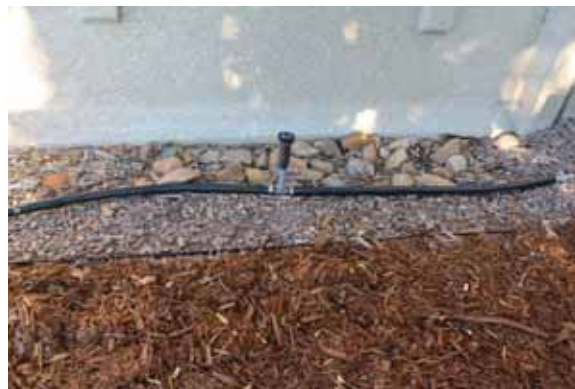
Figure 2.3.B.1 Irrigation along the Building Perimeter
