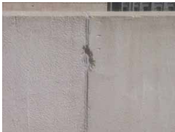
Fig. 2.1.A.7 Spalling at control joint, inside face of roof parapet.
