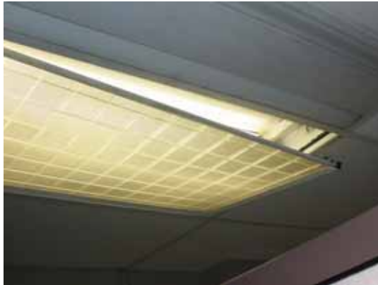
Fig. 2.4.B.3 - Missing panel cover
