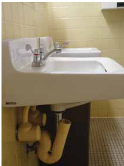
Fig. 2.1.C.2 Insulation coming loose around an accessible lavatory pipe.
