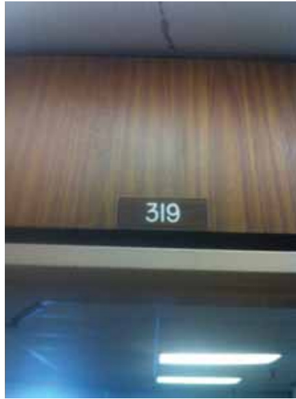
Fig. 3.3.C.1 Damaged 2x4 acoustic ceiling tile at Office 319.
