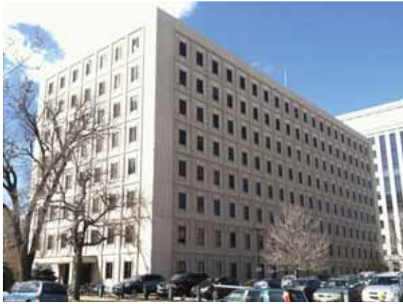
Front & Side/East & North elevation of the Centennial Building
