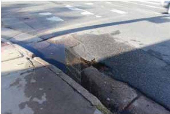
Figure 2.3.B.2 Localized Ponding
