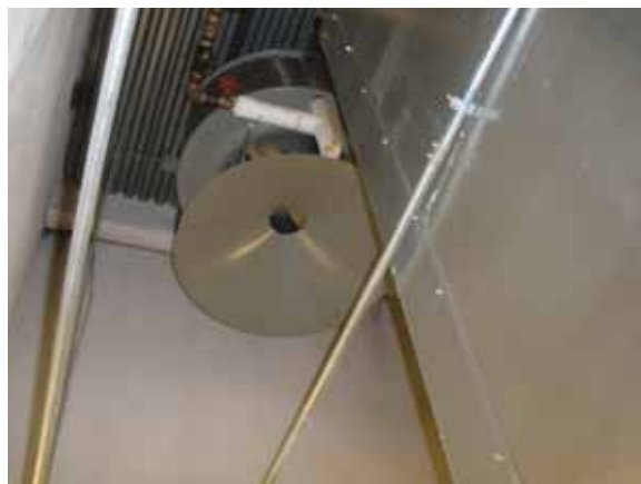
Fig. 2.4.A.9 - Room Unit Heater
